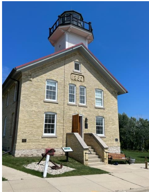
Port Washington 1860 Lighthouse US0114
